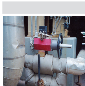
Drum Level Control on a HRSG, provided by a ValvTechnologies' XACTROL®.
